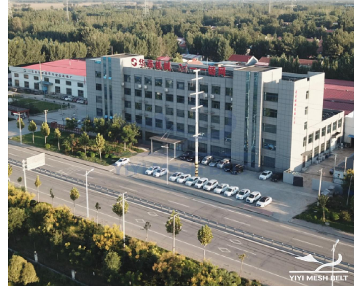
YIYI MESH BELT manufacturing site
