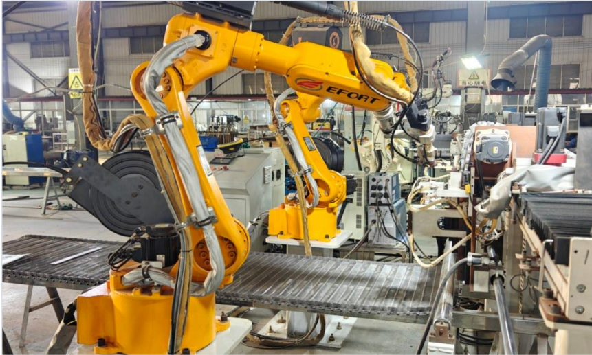
Robot welding cell
